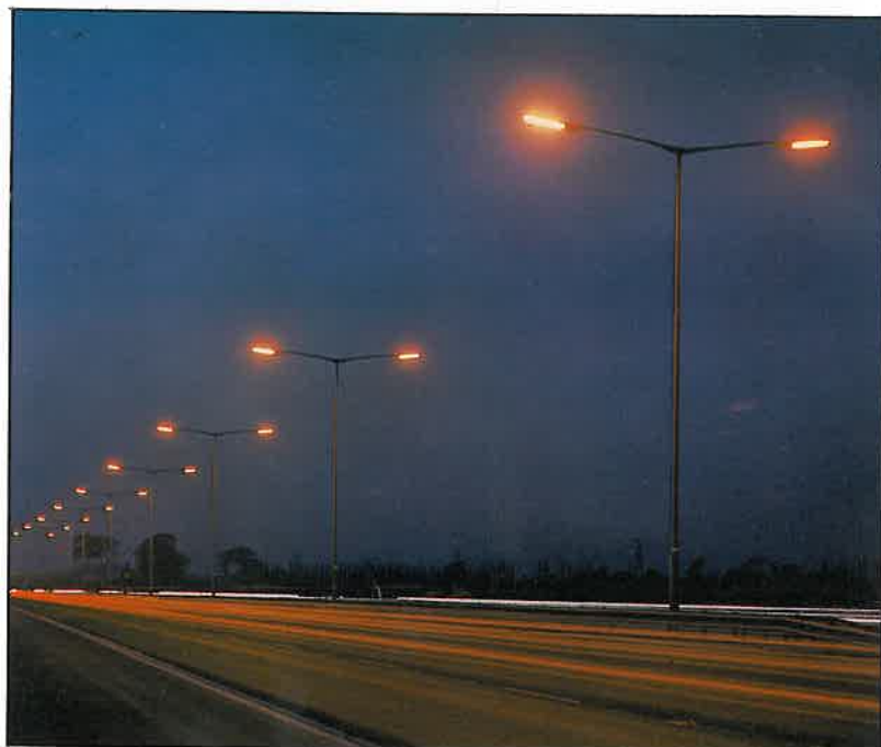
Above Steel rolling mills at Trostre, Wales, lit by high bay discharge lamps. Top Left Spectacular scene a mile inside a north Wales mountain, illuminated by SONline high pressure sodium floodlights. The excavations are for the CEB's Dinorwic pumped storage power station at Llanberis. Left Section of motorway near Coventry illuminated by low pressure sodium lamps.
